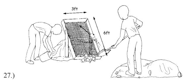
Sift the gravel by throwing the unsifted dirt at the top of the screen. As the gravel falls to the bottom, the proper mix size will fall through.
