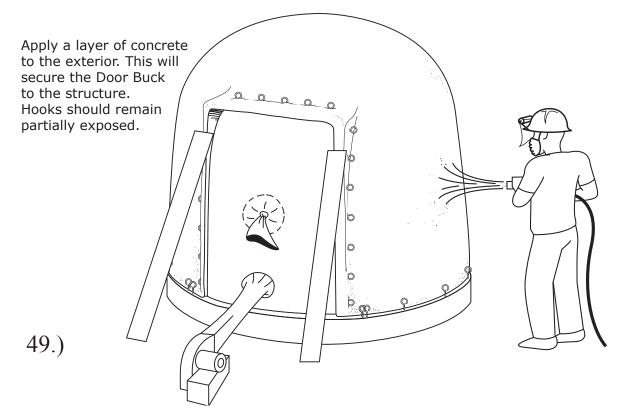
After the primer is added, apply a thin first layer of 1/2" concrete. Once first layer is set, spray on a second 1/2" layer. The 1" thick concrete should completely and evenly cover the Airform while uniting the augmentation(s) to the EcoShell. Here, the first layer of concrete is being added using a Shotcrete pump.
