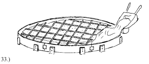
Mix concrete for the floor, by hand if you like. Concrete should be placed fast enough to prevent cold joints. Keep putting fresh concrete against older concrete all the way around.
