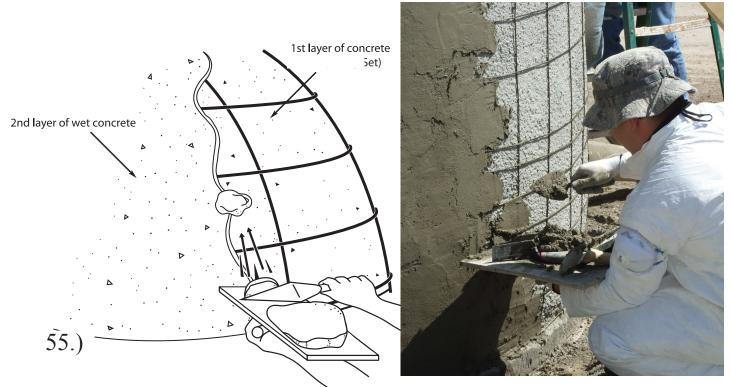
Apply the final layers of concrete using a hand trowel or shotcrete pump.
